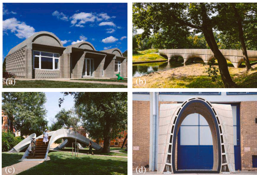
Fig. 1. 3D printed showcases: (a) Wujiazhuang farmhouse, China [11]; (b) Nijmegen bicycle bridge, Netherlands [12,13]; (c) Striatum bridge, Italy [14,15]; (d) Shell pavilion [16].
