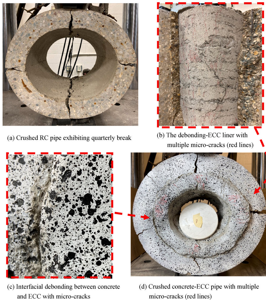
Fig. 20. Crack patterns of the RC-ECC pipe.
