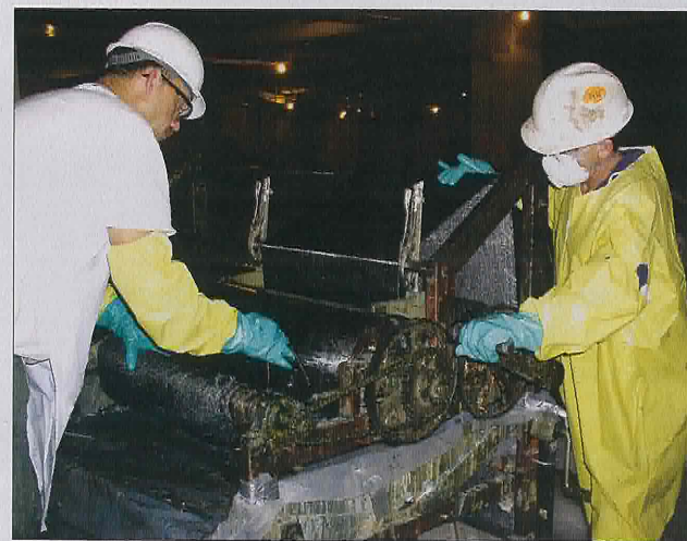
▲ Resin Bath. Epoxy-coated materials help shore up old structures.
