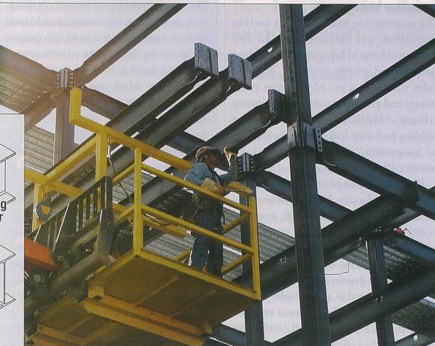
▲ Dovetailed. New moment-resisting space frame (left) slides together quickly (right). Bolts are then added as trades rise through the building.
