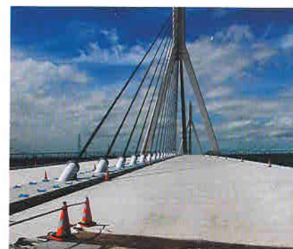
Figure 3: The Mihara Bridge in Hokkaido, Japan, with an ECC/steel deck.
