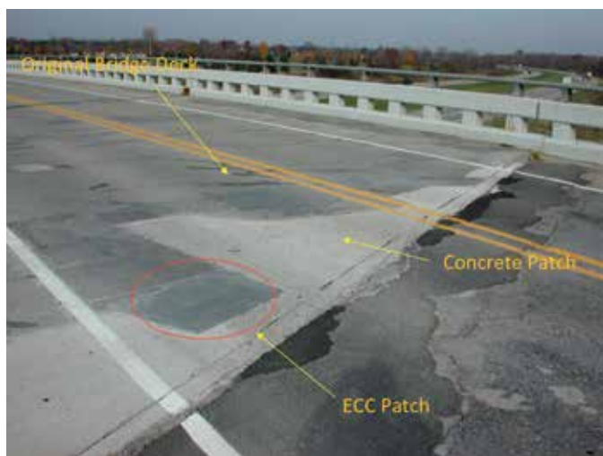
Fig. 7: ECC patch repair placed alongside concrete patch on Michigan bridge deck
