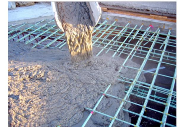
**Figure 7** Self-consolidating ECC enhances quality control in cast on-site projects
