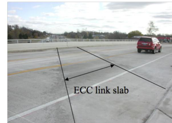
**Figure 6** ECC link slab replaces conventional expansion joints to enhance the service life of bridge deck in the US.
