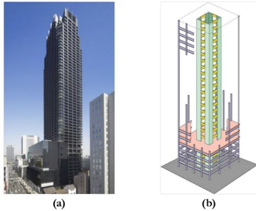
**Figure 9** ECC coupling beams were used to enhance seismic safety in the tallest R/C building in Japan. (a) the 60 story Kitahama Building in Osaka, Japan, and (b) Schematic showing four coupling beams (in yellow) on each floor level.
