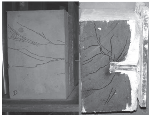
Figure 7. Microcracks developed outside (left) and inside (right, cut section along shear stud) of ECC specimen
