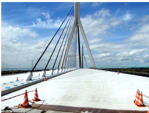
Figure 8: The Mihara bridge (Hokkaido, Japan) uses a steel/ECC composite deck (Courtesy, T. Kanda).
