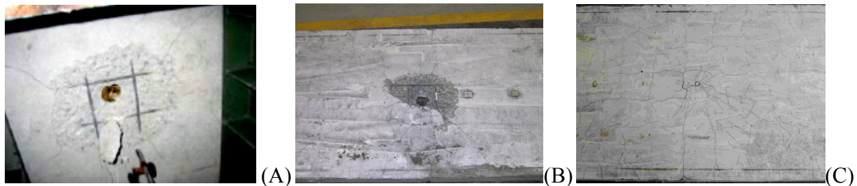
FIGURE 9 - DAMAGE ON DISTAL FACE OF (A) R/C PANEL AFTER 2 ND IMPACT, (B) R/FRC PANEL AFTER THE 7 TH IMPACT, AND (C) R/ECC PANEL AFTER 10 TH IMPACT [ZHANG ET AL, 2005]
