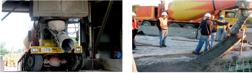
FIGURE 2 - READY-MIX TRUCK MIXING AND SELF-CONSOLIDATING CASTING OF ECC
