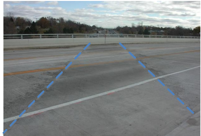
Figure 15 Bridge deck showing ECC link-slab (between dashed lines) after bridge re-opened to traffic
