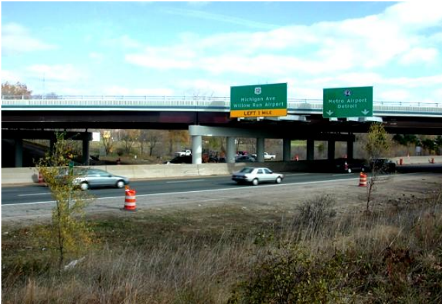
Figure 14 Application of ECC on deck retrofit of a highway bridge in Southeast Michigan
